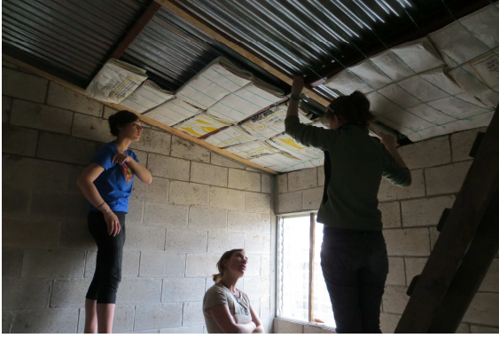
Installation of Insulation
